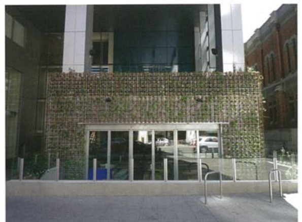
Perth’s permanent Greenhouse cafe. Photo: Tone Wheeler
